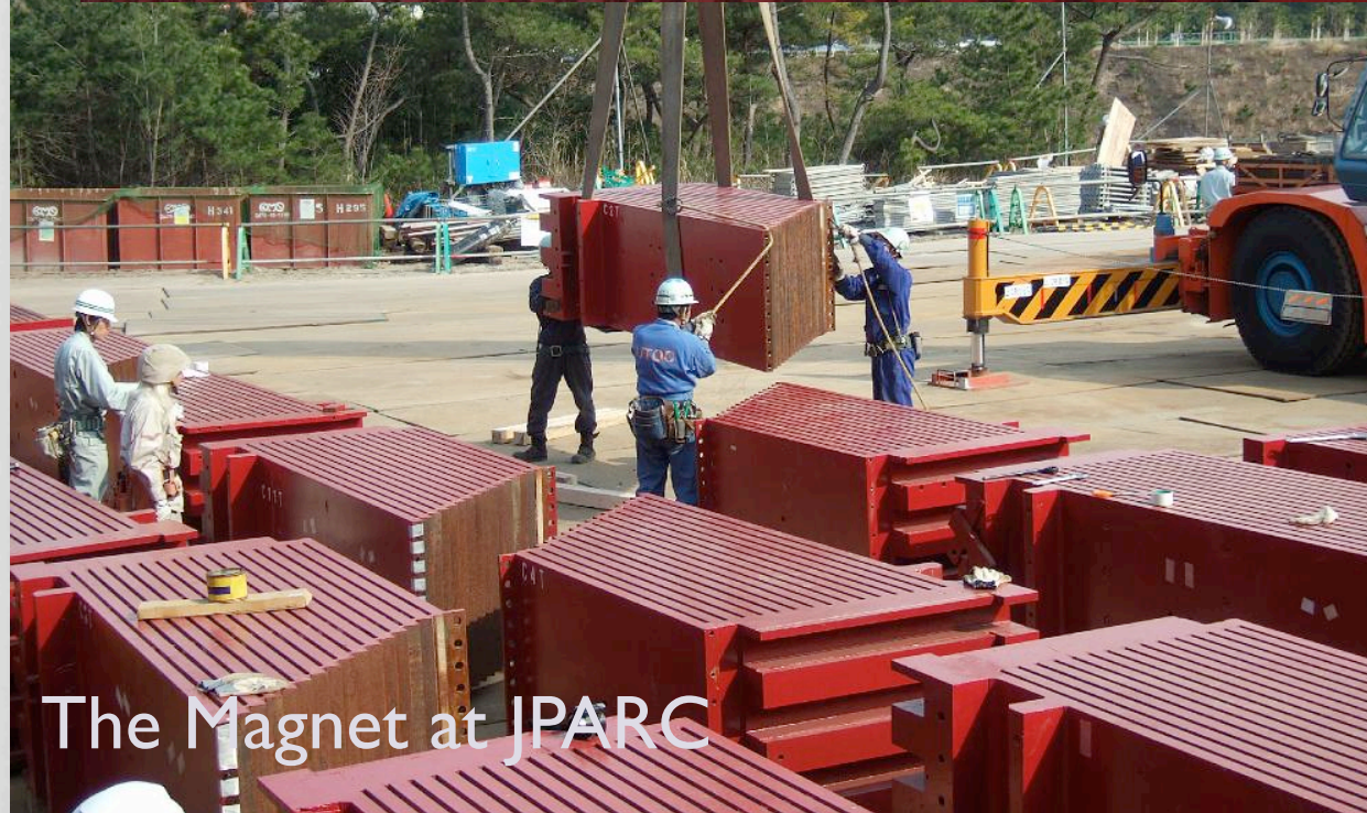
Installation of the coils
